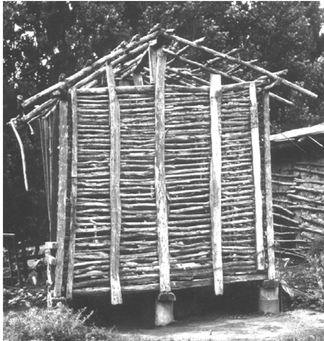
Fig. 7. A construction raised on logs from Ialomiţa County.
